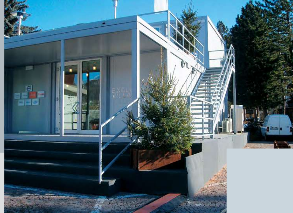
steel frame buildings
